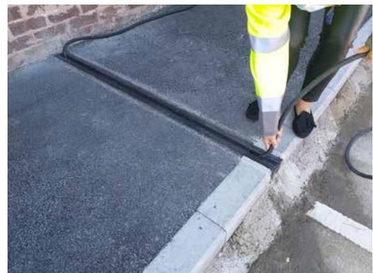
**Figure 27: OxGul-e cable channel**
