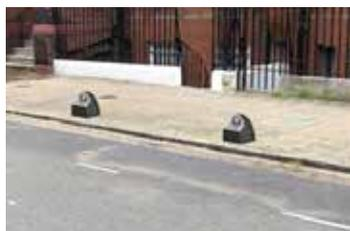
**Figure 14: Connected Kerb Armadillo kerbside charge point**
