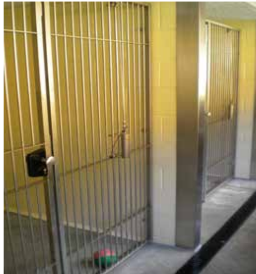
Drainage and building materials
