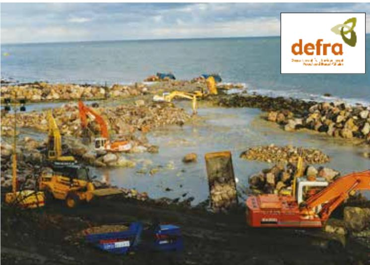
*The Western Cliffs along the Ventnor Undercliff (above) are composed of reconsolidated landslide debris. Aggressive erosion can destabilise clifflines with the risk of promoting further instability, which would adversely affect development on the landslide benches behind. In an attempt to reduce coastal erosion along these cliffs rock protection was provided in 1992.*
