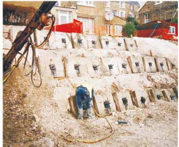
*Soil nailing the upper slope*
