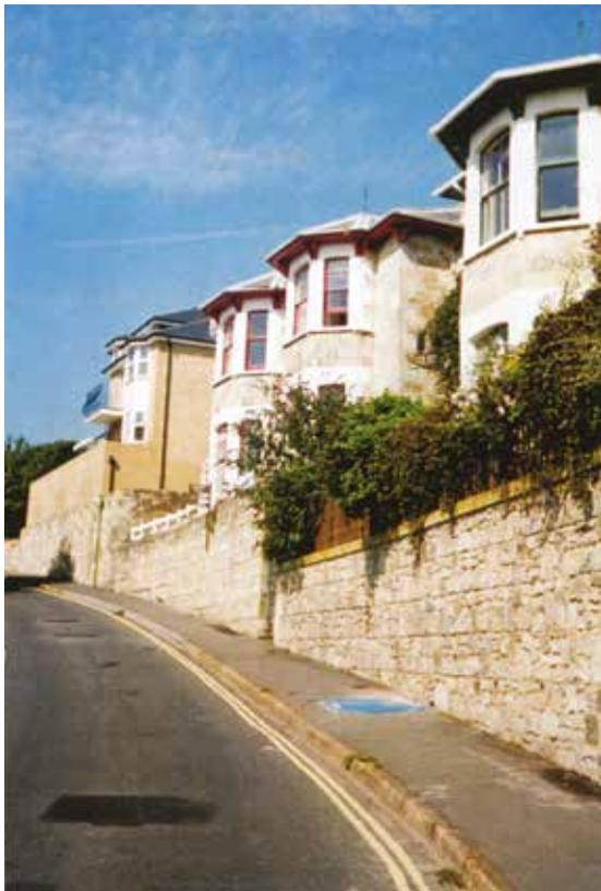
In the case of walls, these may comprise structural retaining walls on suitably designed foundations, sheet or bore piled walls or soil strengthening measures, for example ground and rock anchors or soil nails which may be pre-stressed.
