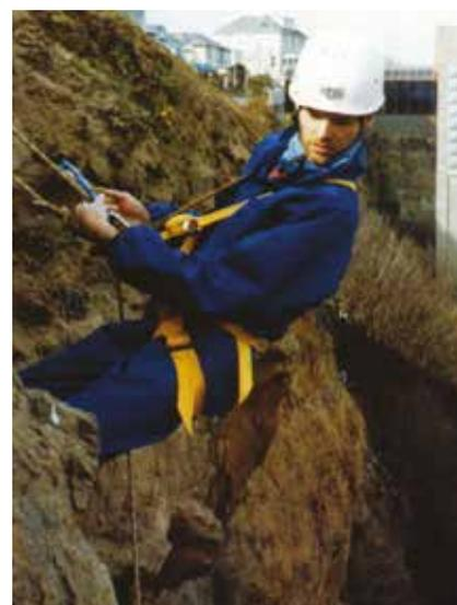
*Cliff face inspection being undertaken by abseiling. Recorded survey data assists in updating the cliff risk assessment*
