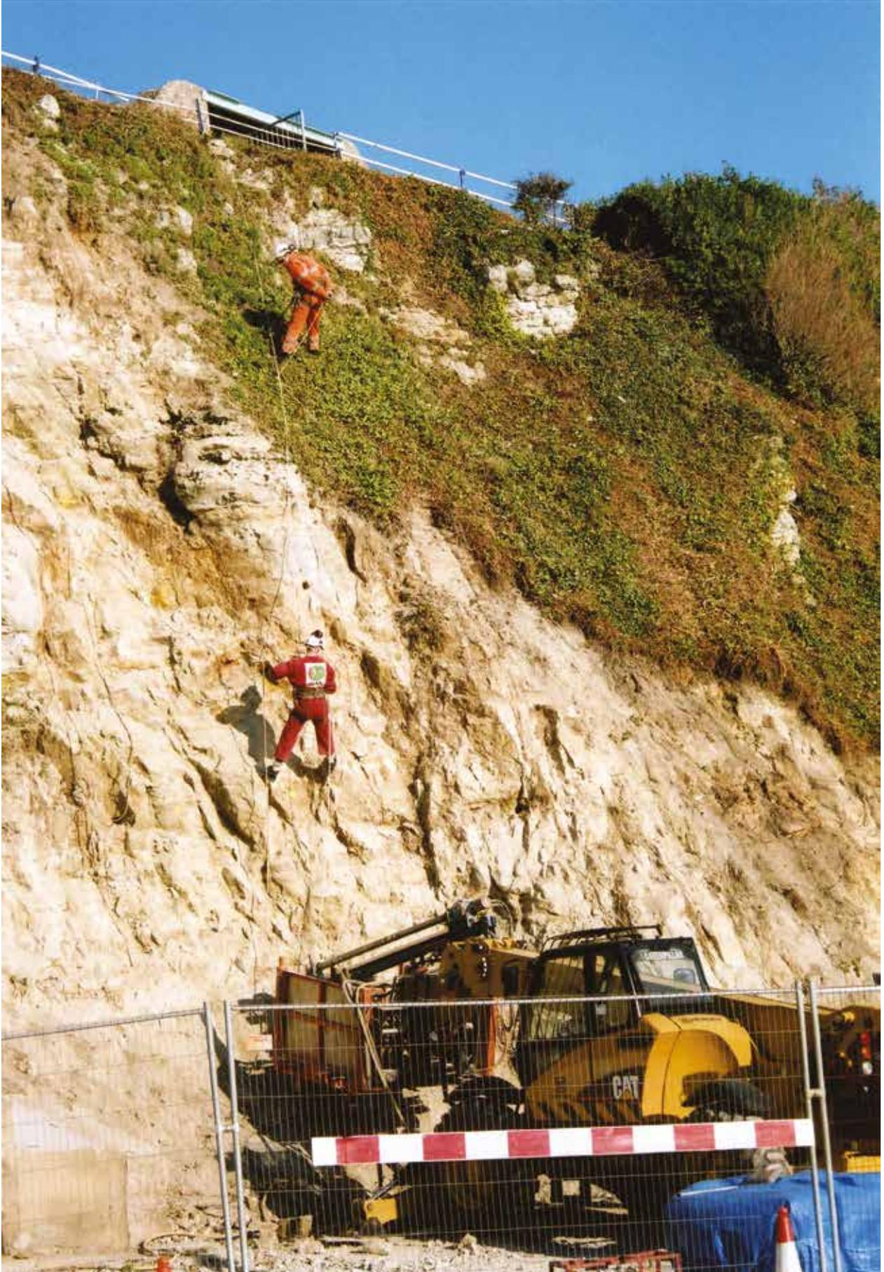
*Reducing rockfall hazard by scaling, bolting and netting at Ventnor Eastern Cliffs - Spring 2006.*
