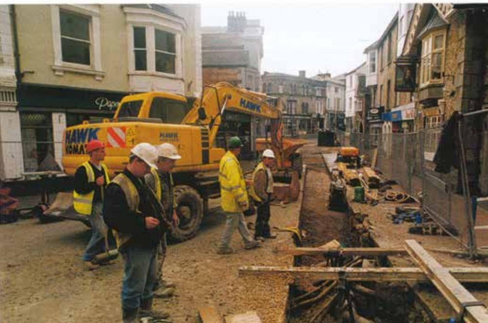
Sewer laying by Southern Water Services Ltd in High Street, Ventnor. The new main was laid through the Undercliff landslide system following a risk assessment of options assisted by geomorphological studies.
