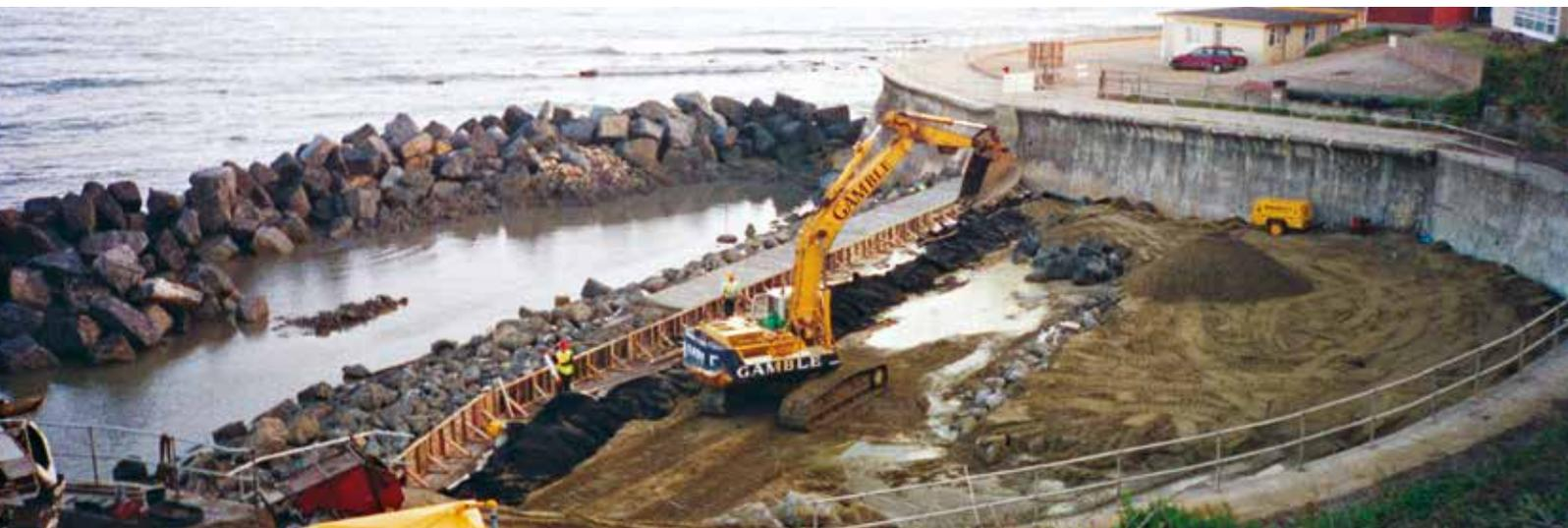
*Constructing the new coastal defences seaward of the existing wall in order to provide support for the slope behind.*
