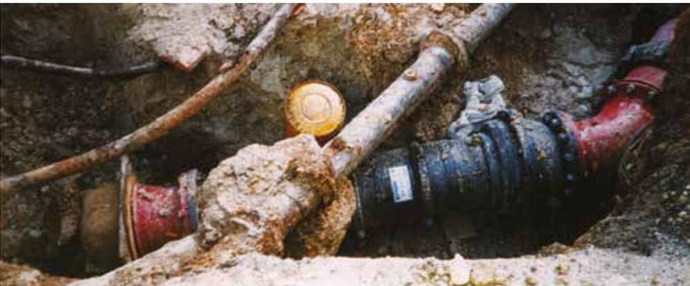
Wherever possible new pipes should be constructed of materials that can accommodate some limited ground movement. This can be assisted by the use of slip joints.
