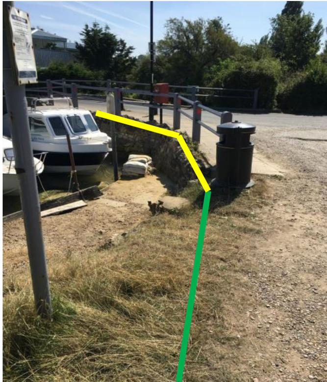
**Photo 9 – Setback Low Earth Bund / Dwarf Wall Required Along a 90m Section of the Frontage Behind the Timber Boards.**
