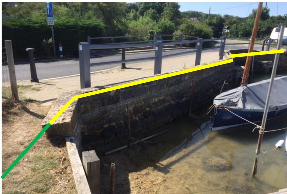
**Photo 8 – Parapet Raising Going into a Setback Floodwall on the Western Side of the Harbour Which Could Run Along the Side of the Access Road and Tie into Defences Towards the Harbour Entrance.**
