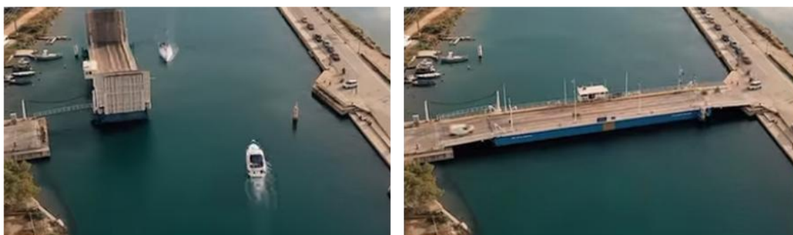
Figure 11. Swinging floating bridge example – Agia Mavra, Greece
