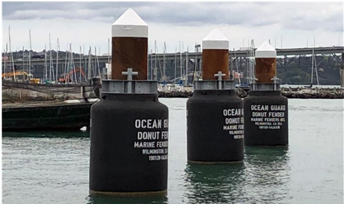
Figure 9. Lead-in piles example
