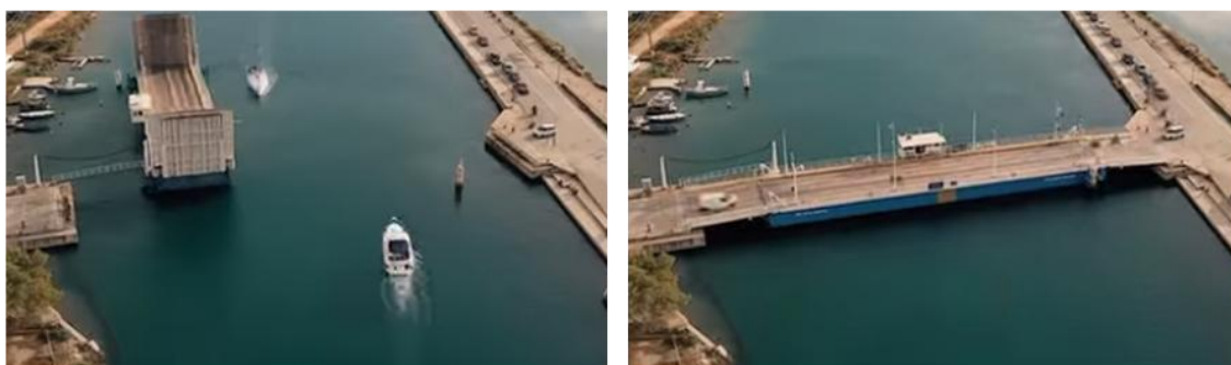
Figure 11. Swinging floating bridge example – Agia Mavra, Greece
