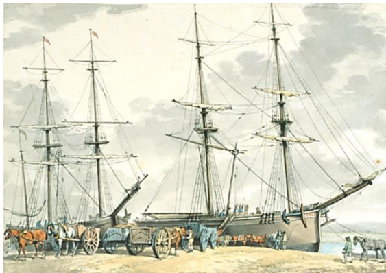
Southampton quay with colliers unloading. IWCMS.2002.68
