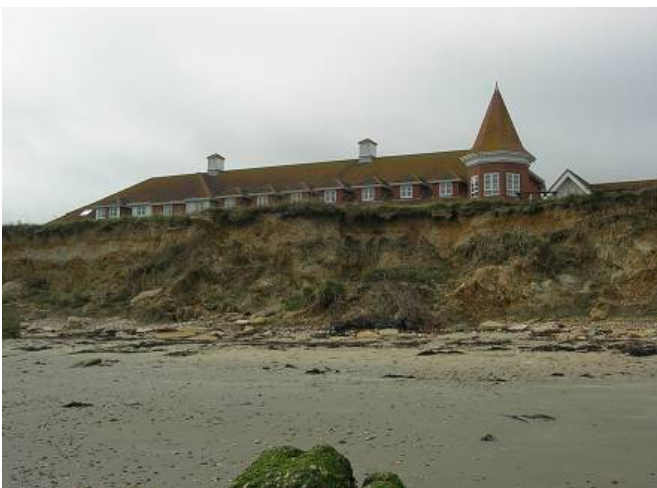
Below: Cliff erosion near Foreland Point
