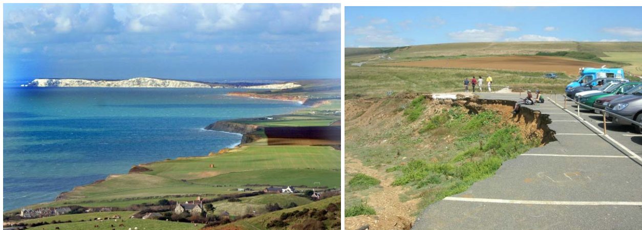
Left to right: View along the eroding south-west coast of the Isle of Wight from near Blackgang in 2009 (N.Dix); Erosion of the car park behind Compton Bay, 2006.
