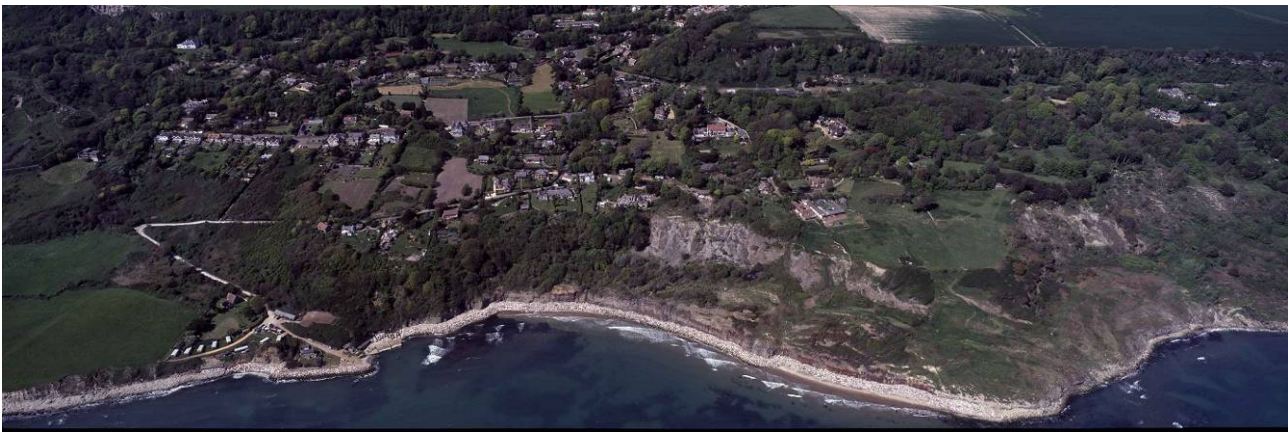
Castlehaven: Reeth Bay rock revetment and slope drainage scheme (Isle of Wight Council)
